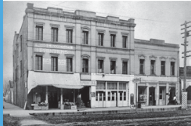
The Holman Building, on the NW corner of Commercial and Ferry streets in Salem, was the location of The Marion-Polk County Medical Society's first meeting. The photo was taken in 1925. (Image courtesy of the Oregon State Library)
